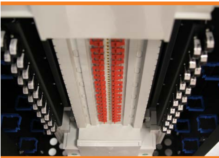
CTs Mounted on a 42-Circuit SafePanel™ Panel Board
