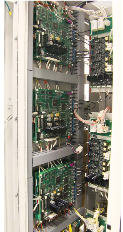
Triple Modular Redundant System Control Boards
