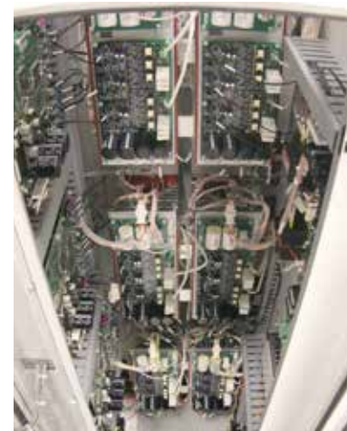
Convection-Cooled Design in an eSTS, showing perforated vents on the cabinet bottom
