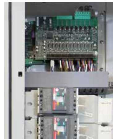
Serialized "Panel Board Monitor" (PBM) in an ePanel-HD2
