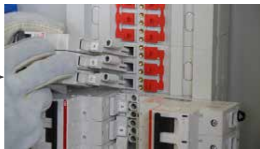
The Breaker Is Inserted Into The Opening
