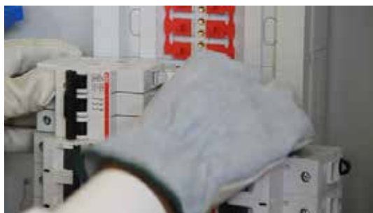
The Breaker Snaps Into The DIN Rail
