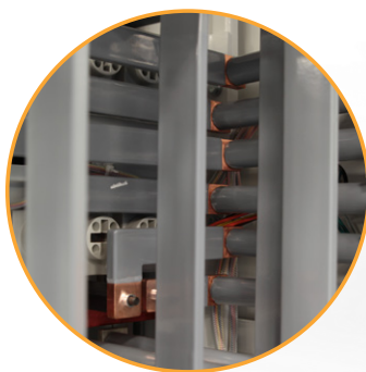
Epoxy helps protect buswork from corrosion, dust, and moisture
