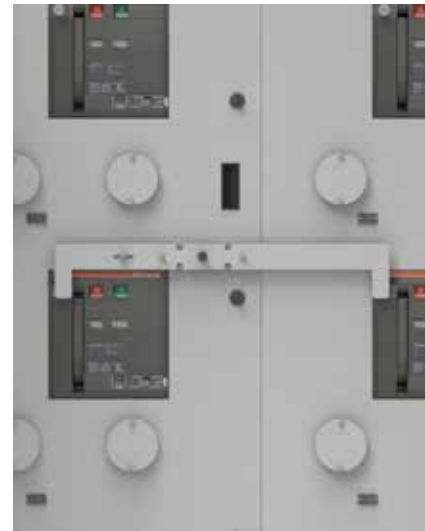
Mechanical Bypass Interlock Design
