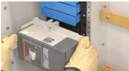
The Breaker Is Inserted Into The SafePanel
