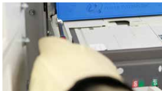
Screws Help Secure The Breaker
