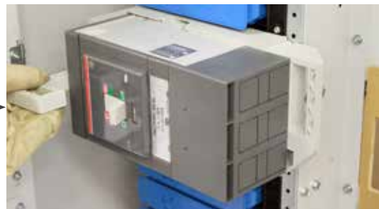
The Handle Is Unlocked
