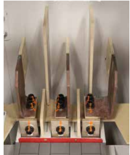
Silver-Plated Customer Connections
