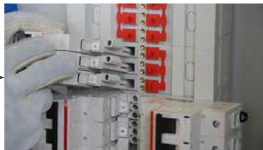
The Breaker Is Inserted Into The Opening
