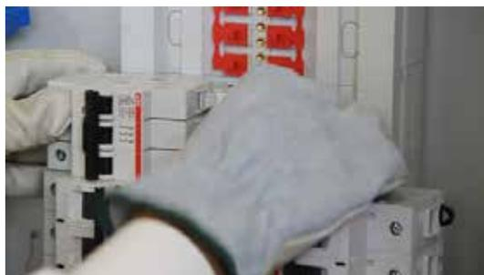
The Breaker Snaps Into The DIN Rail
