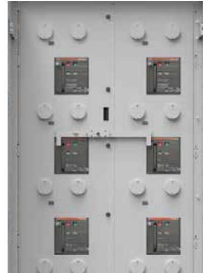
Mechanical Bypass Interlock "Goalpost" Design
