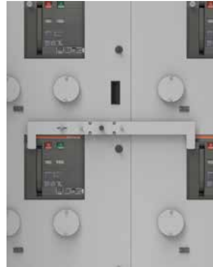
Mechanical Bypass Interlock Design
