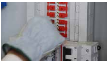
The Protective Cover Is Removed
