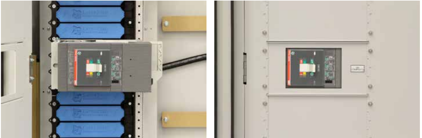
A subfeed circuit breaker installed in the 1200 A SafePanel with a plate on the dead front door installed
