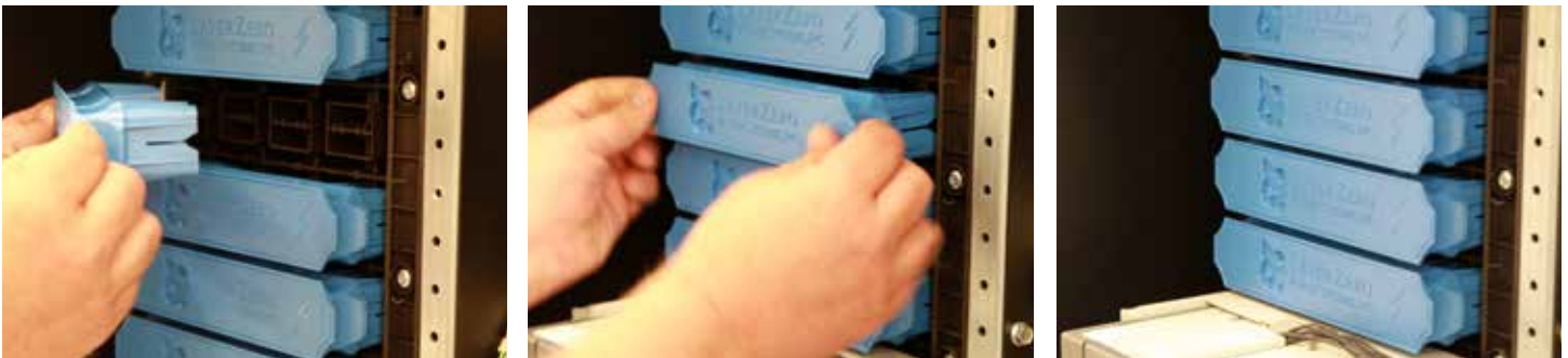
Installation of a subfeed cover
