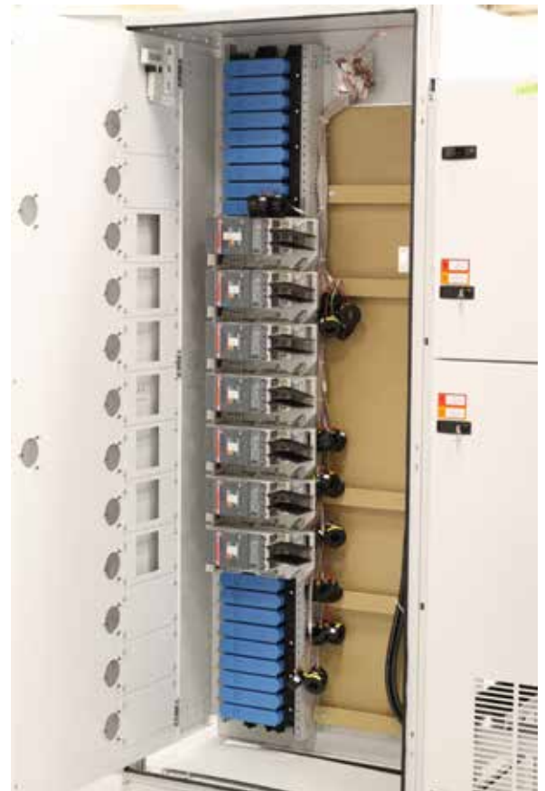
A subfeed circuit breaker installed in the 1200 A SafePanel with a plate on the dead front door installed
