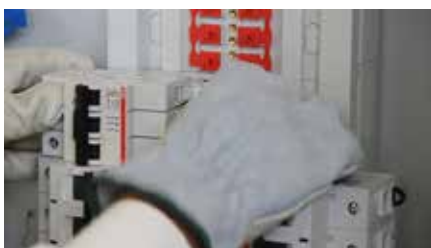
The Breaker Snaps Into The DIN Rail
