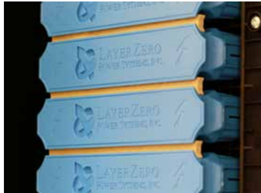
Optional fiberglass link insert in subfeeds
