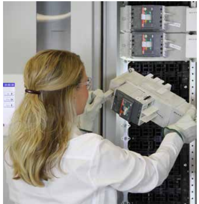
Installing a Subfeed Circuit Breaker in a 1200 A SafePanel
