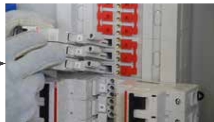
The Breaker Is Inserted Into The Opening
