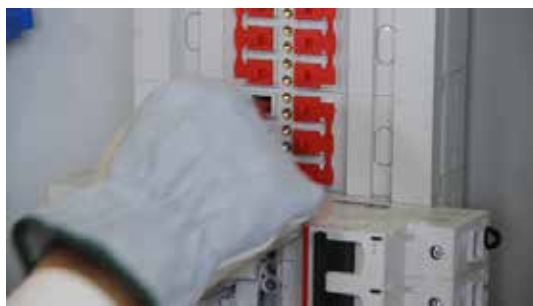
The Protective Cover Is Removed
