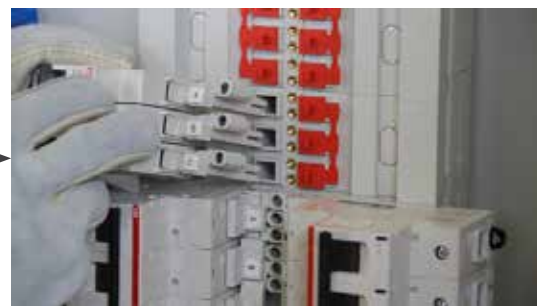
The Breaker Is Inserted Into The Opening
